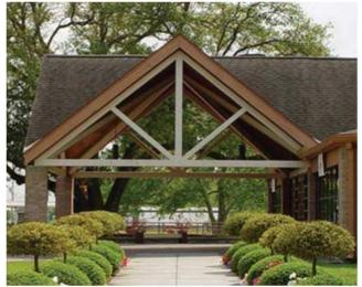
Trusses are commonly used to support roofs.
