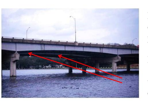
Beams are structural members designed to support loads applied perpendicularly to their axes.
