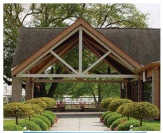
Trusses are commonly used to support roofs.
