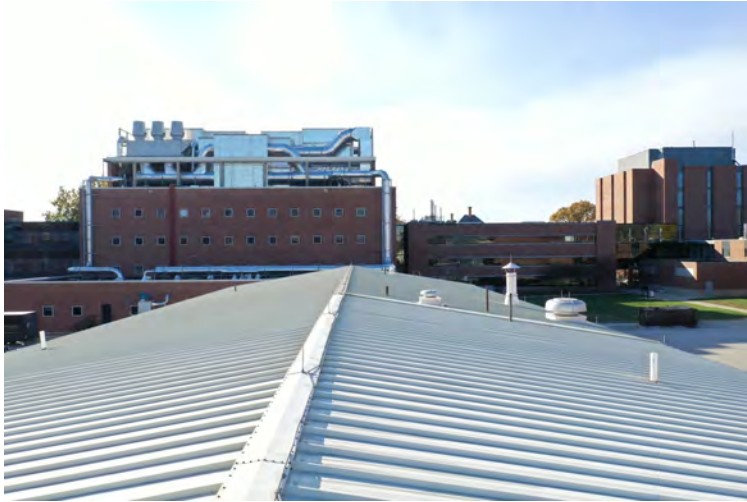
(a) Aerodynamics Research Building Rooftop
