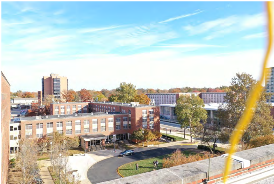
(d) Northwest Corner of Loomis Laboratory Rooftop Facing Southeast
