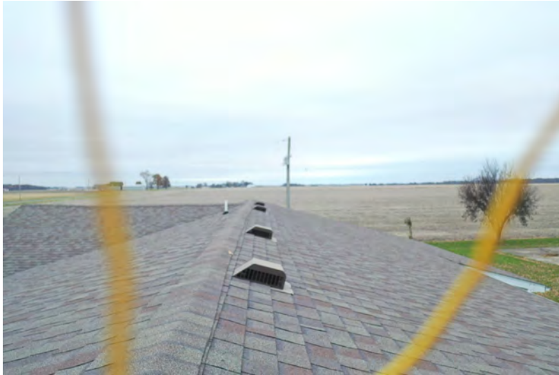
(c) Farmhouse Rooftop With Heat Vents (431 County Rd 700 N Sadorus, IL)
