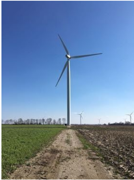
Figure 3: Wind Turbine at location 40.203677, -87.875488.
