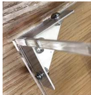
Figure 22: Angle Bracket Fixing between Acrylic Panels
