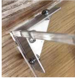
Figure 23: Angle Bracket Fixing between Acrylic Panels
