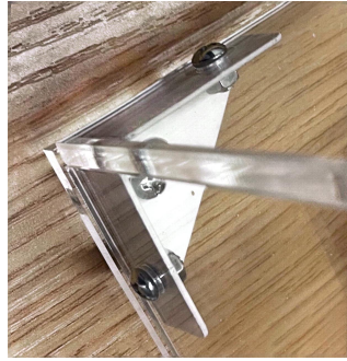
Figure 18: Angle Bracket Fixing between Acrylic Panels
