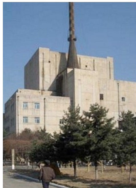
Reactor, Yongbyon, NK
