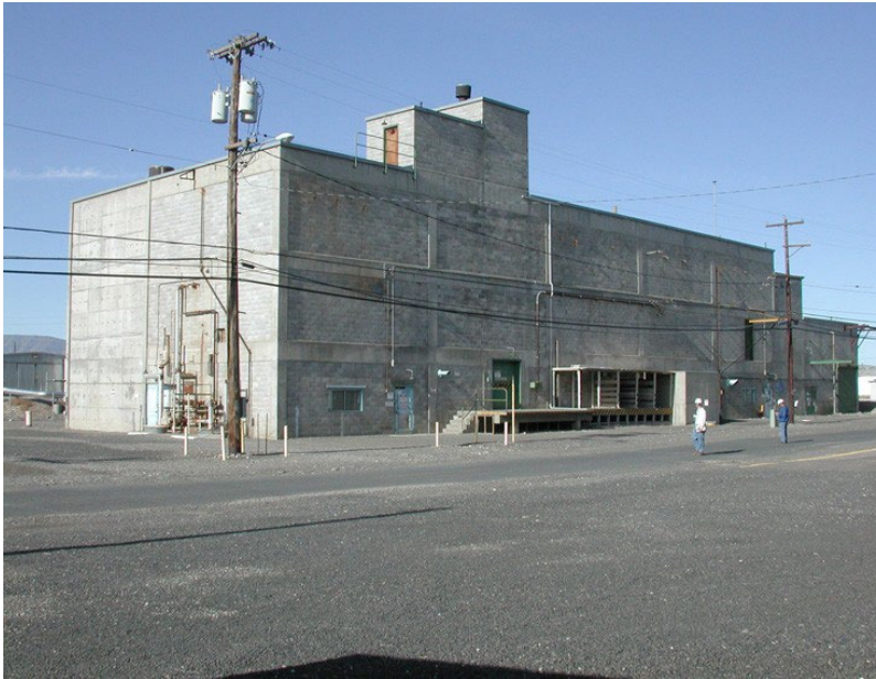
224-B Plutonium Separation Plant, Hanford, WA, 1985
